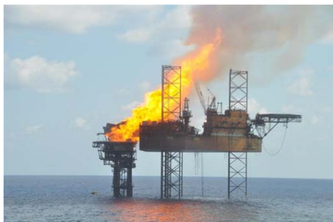
The Montara oil rig on fire on 2 November. Photo courtesy PTTEP Aust
